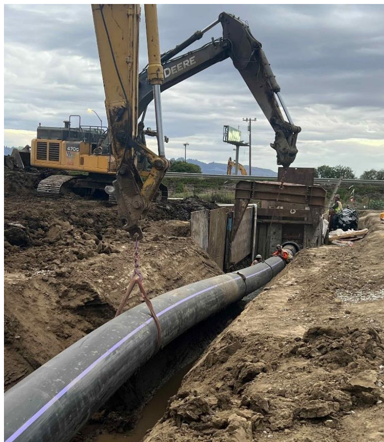
College Lake Water Supply Pipeline being thread under Highway 1, Nov.15, 2023
