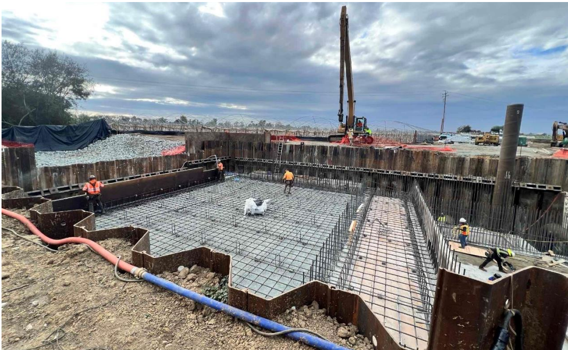
College Lake Water Supply Project Weir and Pump Station Construction: Fall 2023
