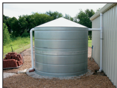
2,500 Gallon Catchment Tank
