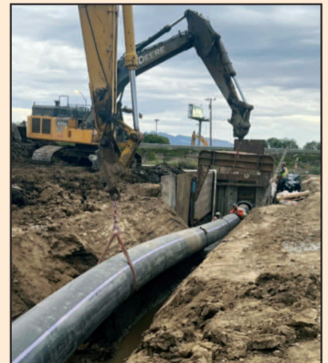
College Lake Water Supply Pipeline being thread under Highway 1 Nov. 15, 2023
